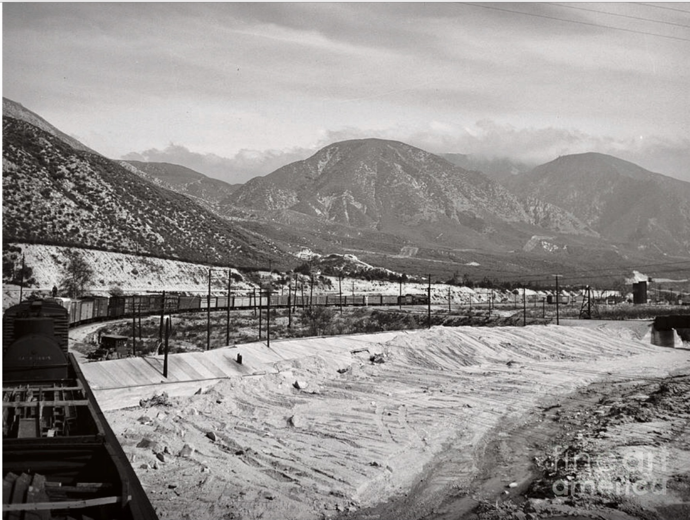
1944 Delano Photo? Shows revetment between bridges east of Cajon Station Creek bottom appears to have be recently bulldozed.
