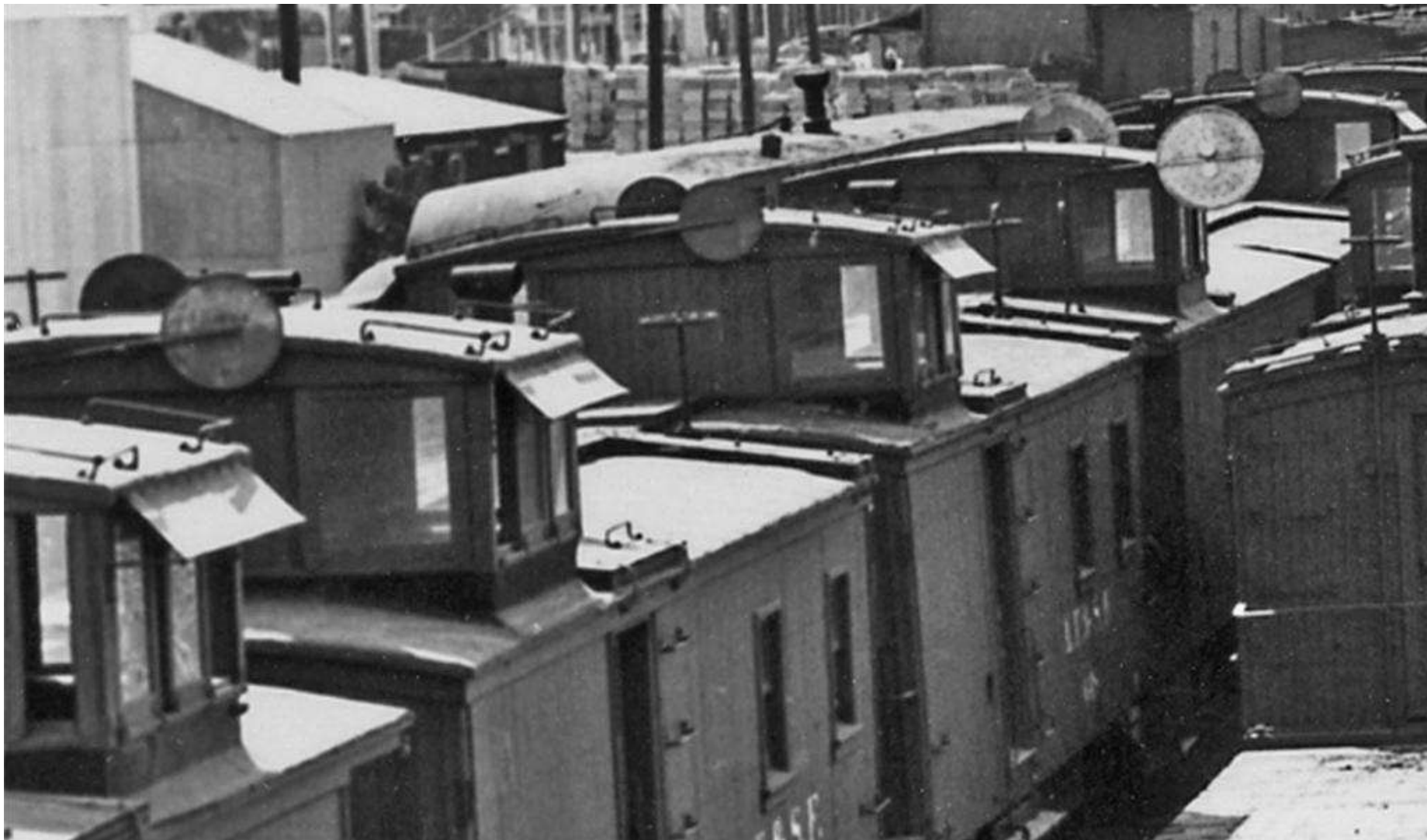
La Junta wig-wags on wooden cabooses Wig-wags style 1 and style 7 show up on side door wood cabooses
