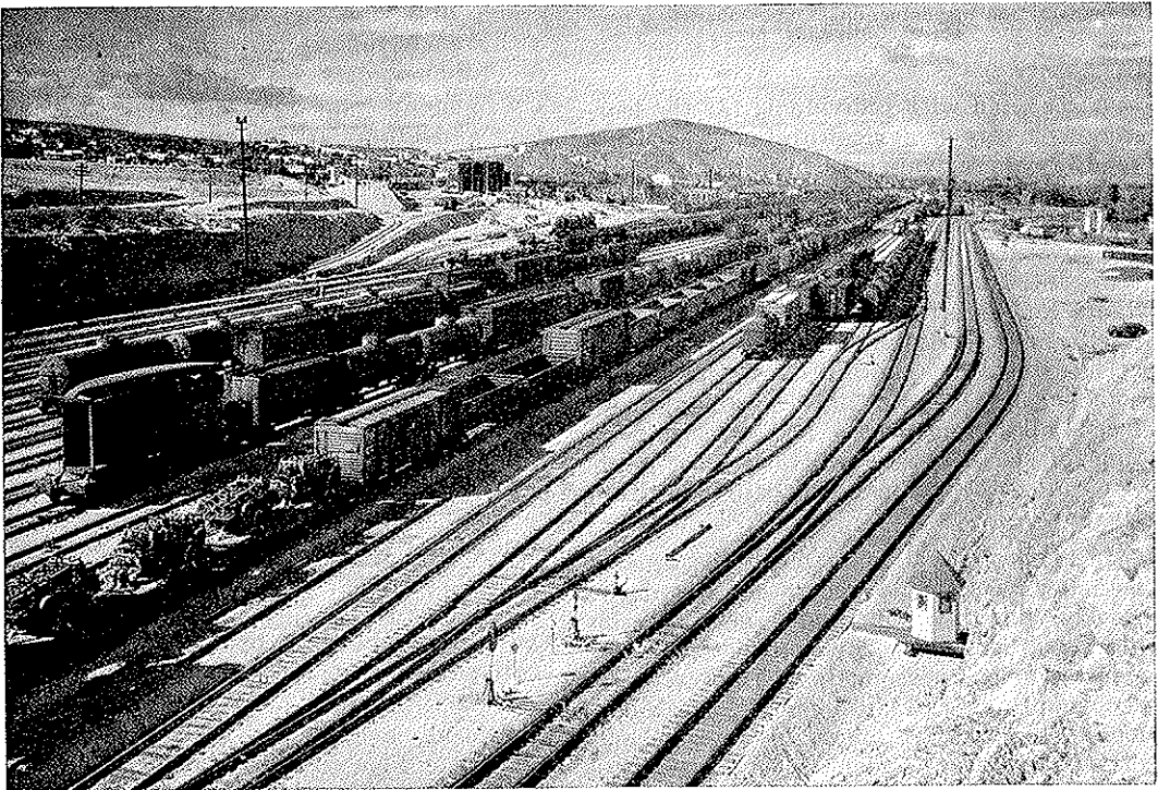
IMPORTANT CONSOLIDATION YARDS, such as at Barstow (above), are natural converging points for hundreds of cars of freight. At such places trains are broken up, cars are switched and new trains are made up as efficiently as possible to speed the railroad's traffic on its way with the least amount of delay and interruption.
