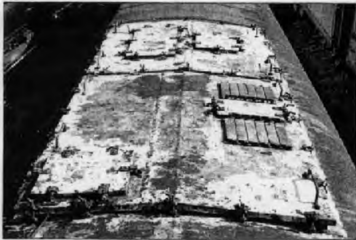
Roof hatch detail on San Bartolo (ex 1363 a lounge/dorm) at Fair Park in Dallas. Note air duct on right. Both a/c and refrigeration hatches on end of car. There is a slight variation between the a/c hatch on this car and 3231 to the right.
