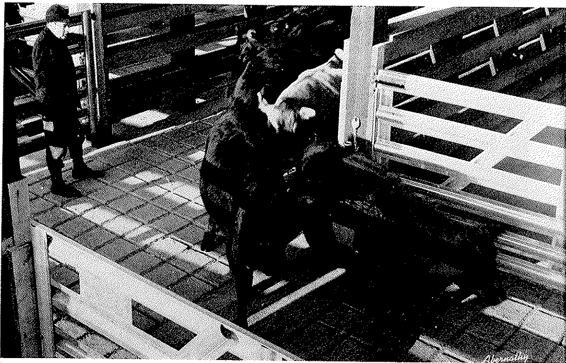
Non-Slip Concrete Paves Alleys
